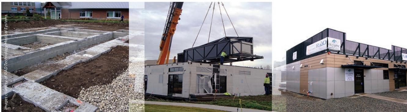
Patented foundation and shielding systems made the modular temporary radiotherapy vault economical to ship and quick to install.
